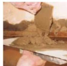
**PLANITOP 450: MORTIER D'ASPECT FIN ET CLAIR, THIXOTROPE, FRIBRÉ ET À RETRAIT COMPENSÉ**
