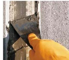
**MAPEFLEX PB25: MASTIC POLYURÉTHANE BICOMPOSANT, THIXOTROPE, À BAS MODULE ÉLASTIQUE, RÉSISTANT AUX HYDROCARBURES**
