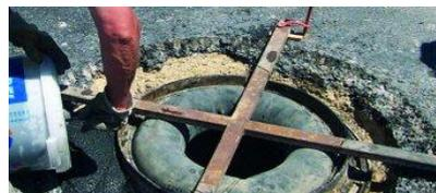
**MAPEGROUT SV T GRAVIER: MICRO-BÉTON THIXOTROPE DESTINÉ À LA RÉPARATION ET AU SCELLEMENT D'ÉLÉMENTS DE VOIRIE**
