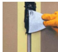
**MAPEFLEX PB27: MASTIC POLYURÉTHANE BICOMPOSANT, COULABLE, À BAS MODULE ÉLASTIQUE, RÉSIDANT AUX HYDROCARBURES**
